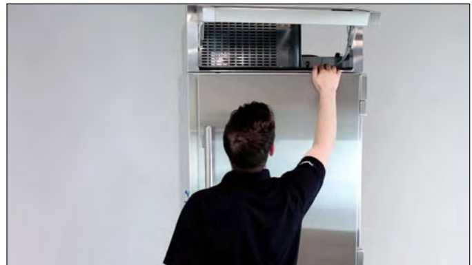
FIG. 3. Be sure to inspect behind the rainshield.
