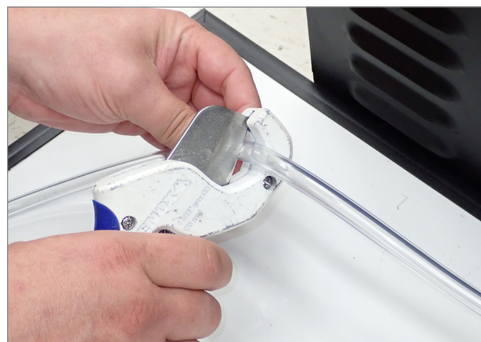
FIG. 3. Cut the drain line with tubing cutters.
