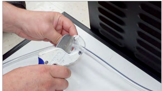
FIG. 3. Cut the drain line with tubing cutters.
