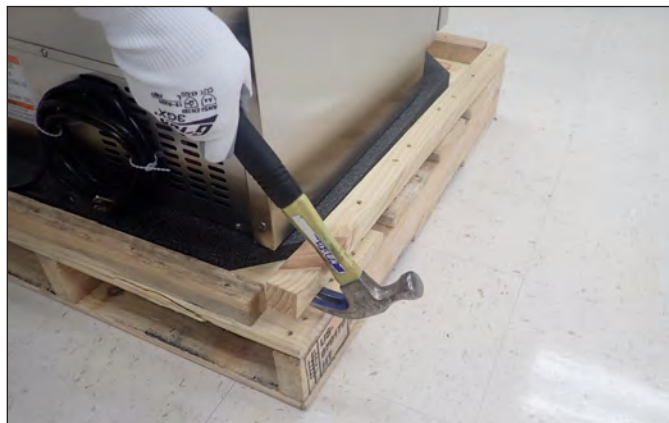
FIG. 2. Pry the side runner board off the skid.
