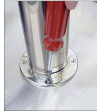
FIG. 3. Secure the draft standard to the countertop.
