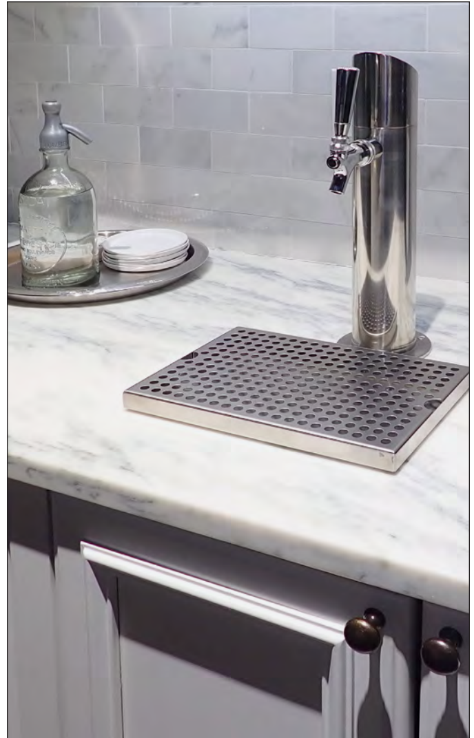
FIG. 1. Example of countertop draft standard installation.
