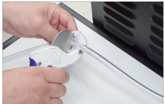
FIG. 3. Cut the drain line with tubing cutters.
