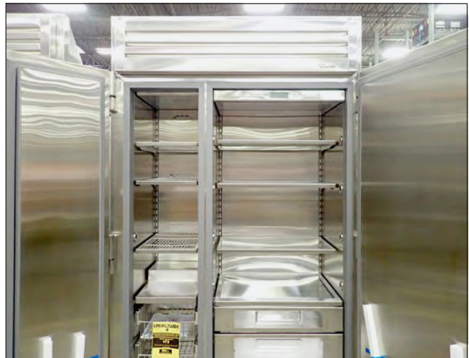
FIG. 7. Completed shelf installation.
