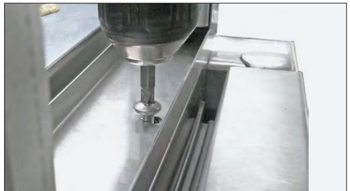
FIG. 10. Remove the screws from the metal channel.
