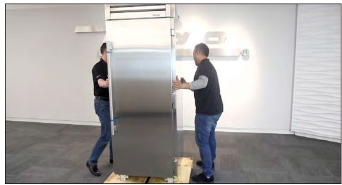
FIG. 10a. With assistance, carefully walk the appliance partially off the back of the skid.
