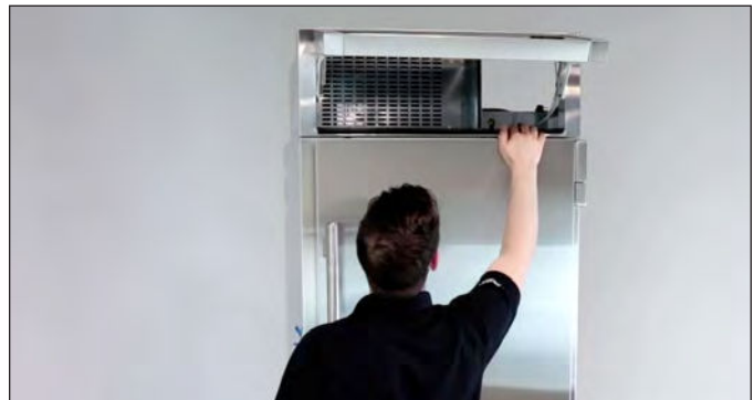
FIG. 3. Be sure to inspect the rainshield.
