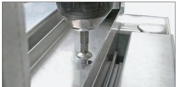
FIG. 10. Remove the screws from the metal channel.
