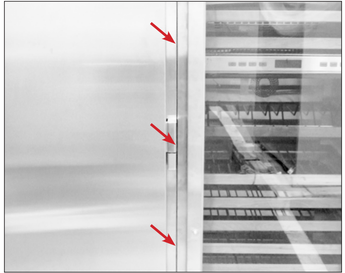
FIG. 16. Verify the gap(s) between appliances is (are) even throughout.
